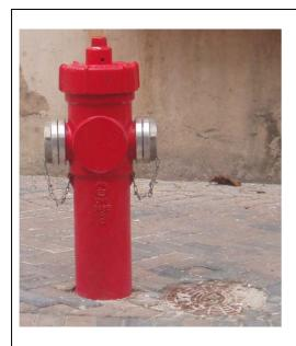
Fire hydrants should meet the specifications of the Fire Department. The hydrants should be fitted with a 2½ Storz (German) connection as specified per DIN 3222. The hydrants should be placed above ground. The Storz connection must be covered by a blind Storz cover that is attached to the hydrant by a chain.
